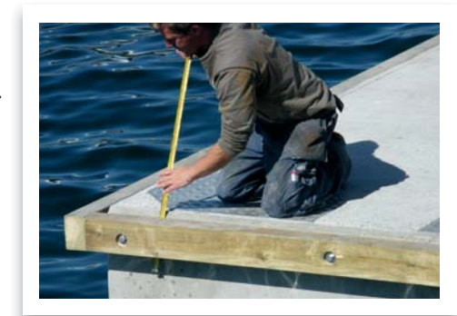
Measuring pontoon freeboard
