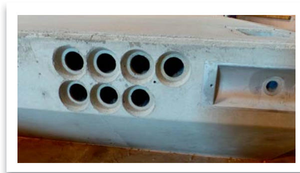
Ducts for water and electricity
